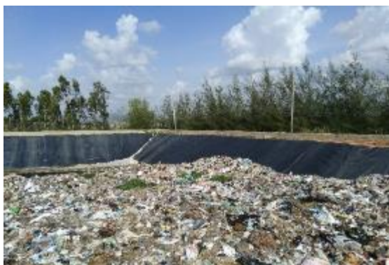
Sanitary Landfill facility at the dumpsite
